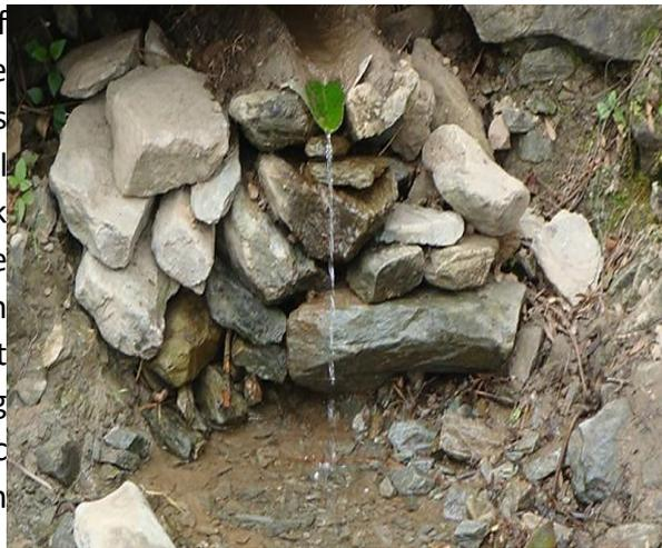
*Figure 4: Channelization of spring*
