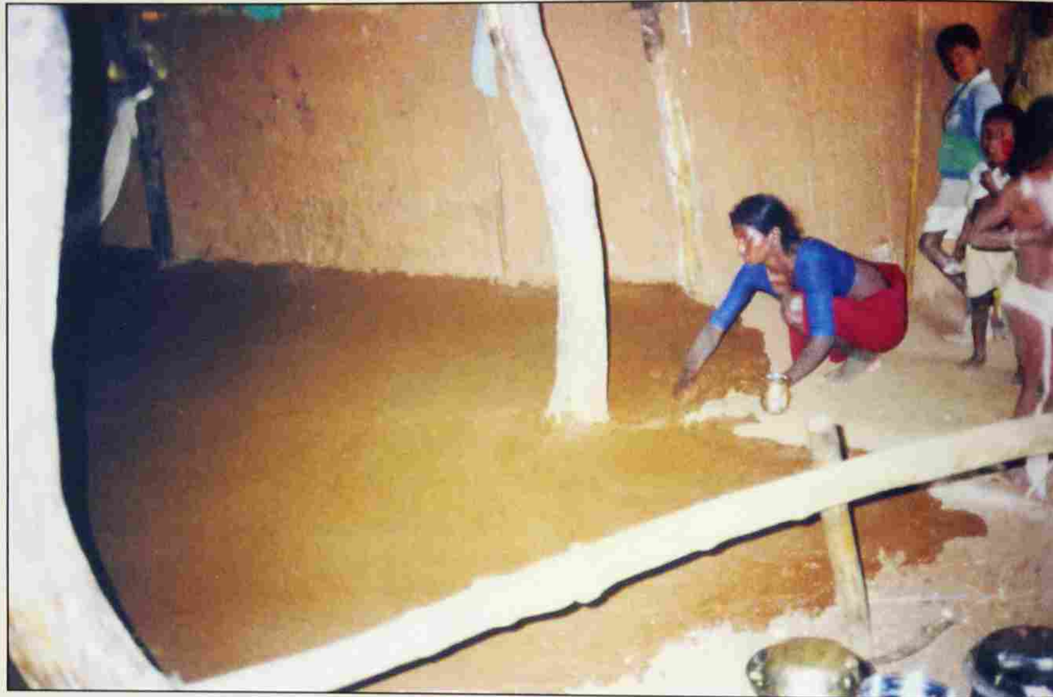
Plastering the floor
