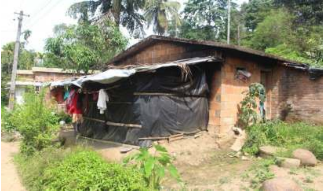
Picture 11 to 14. Conditions of houses in different Paniyan settlements in Wayanad
