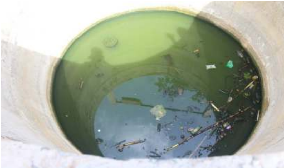
Picture 21. Contaminated well in the tribal settlement
