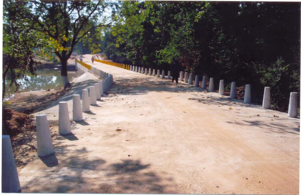
Construction VCW at Naraharibagicha
