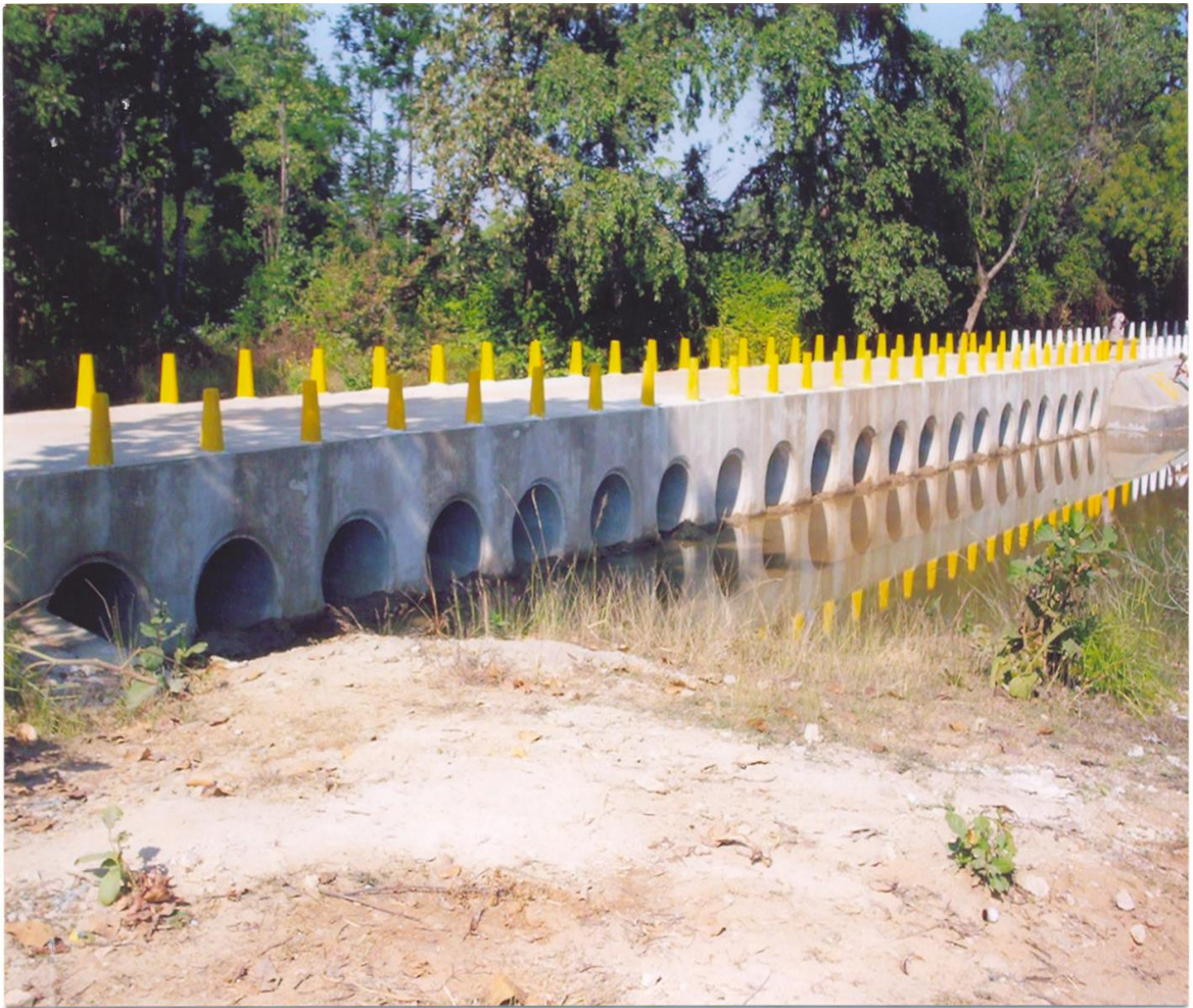
Construction of V.C.W. at Naraharibagicha, Kuchinda ITDA
