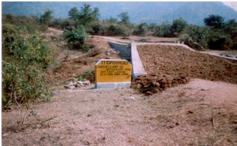
Cross Drainage Work at Sananullah in Kalyansingpur Block (Majhiguda G.P)
