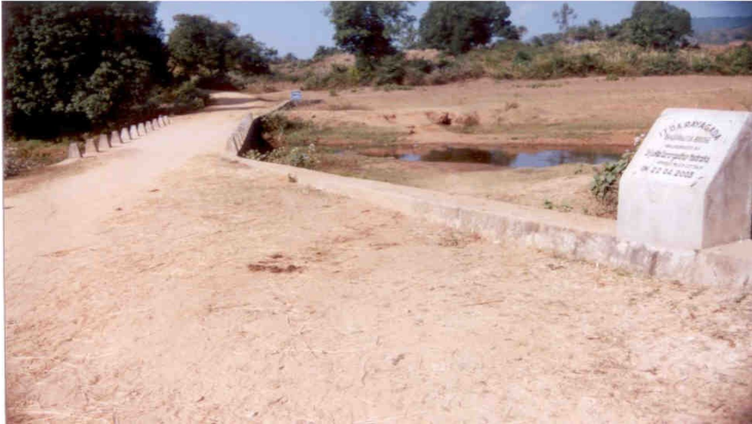
Cross Drainage Work at Matikeswari Road in Kolnara Block (Kolnara G.P)
