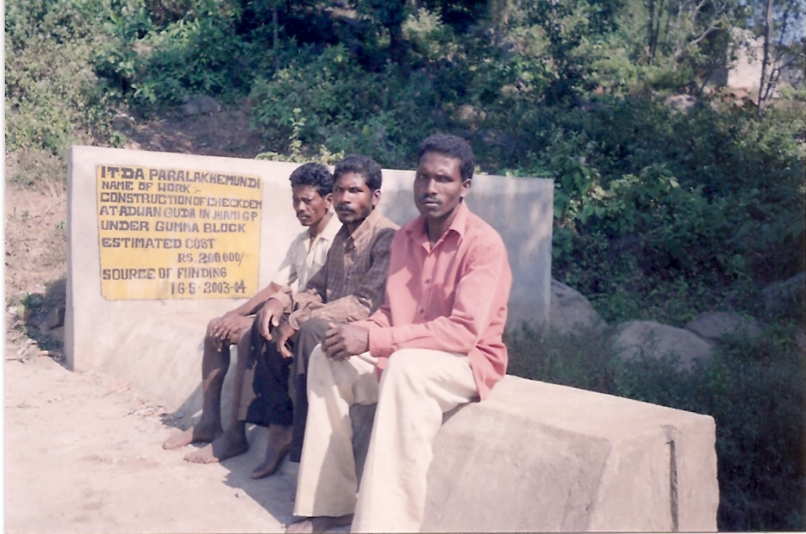
Checkdam (MIP) at Jhala village in Jhamani G.P. of Gumma block
