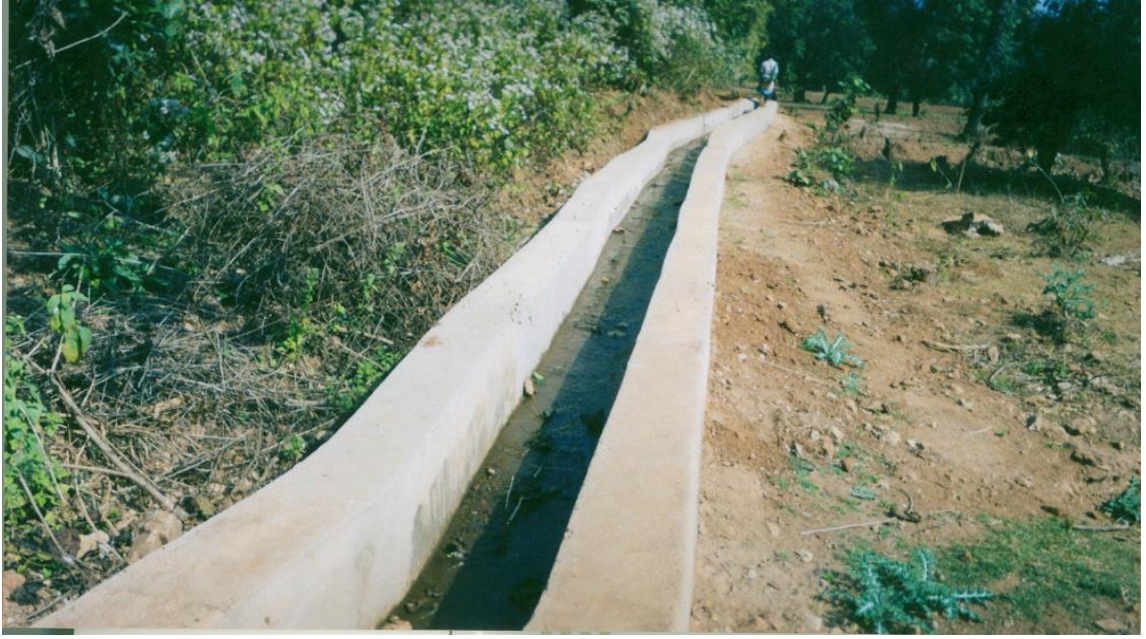
Canal of Pharketa Check dam
