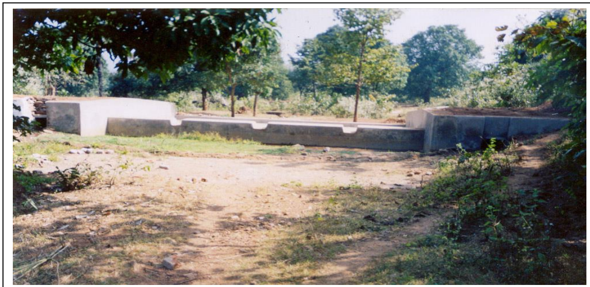
Raigat Nala Check Dam
