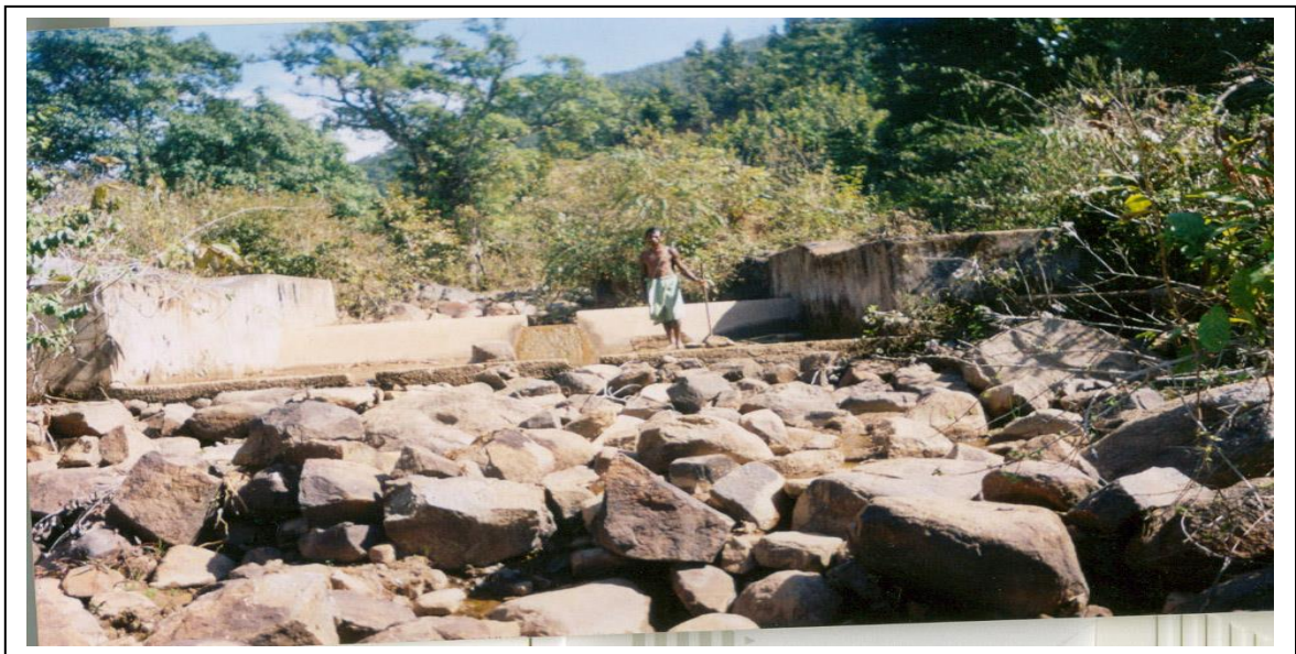
Check Dam at Pinga Suga Nala
