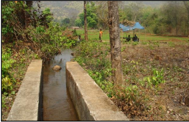
Budhigaon Diversion Weir on river Deo in Karanja Block
