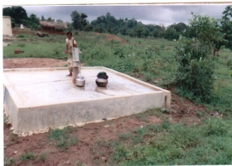
Piped Water Project at Khejuri village, DKDA, Kurli, Chatikona
