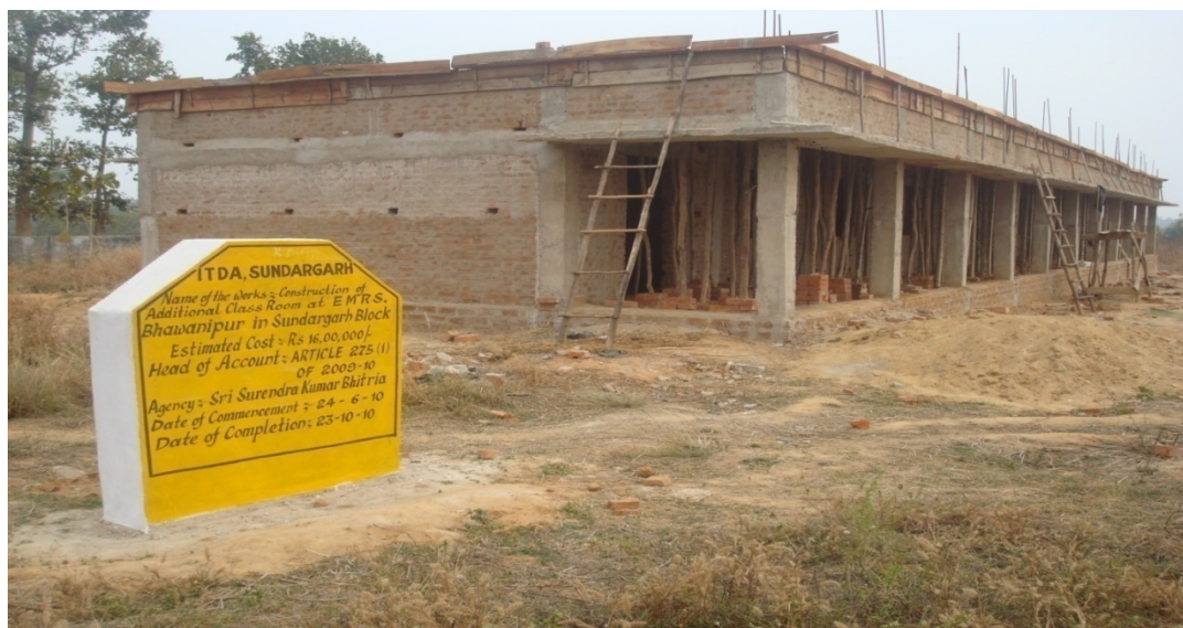
Class rooms of the EMRS are under construction
