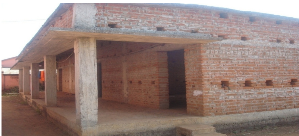
Class Rooms are under construction
