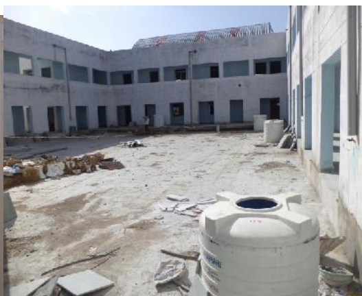
Hostel Construction in EMRS Narainala
