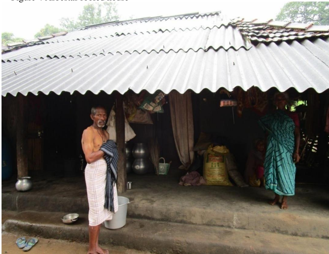
Figure 4 Asbestos roofed house
