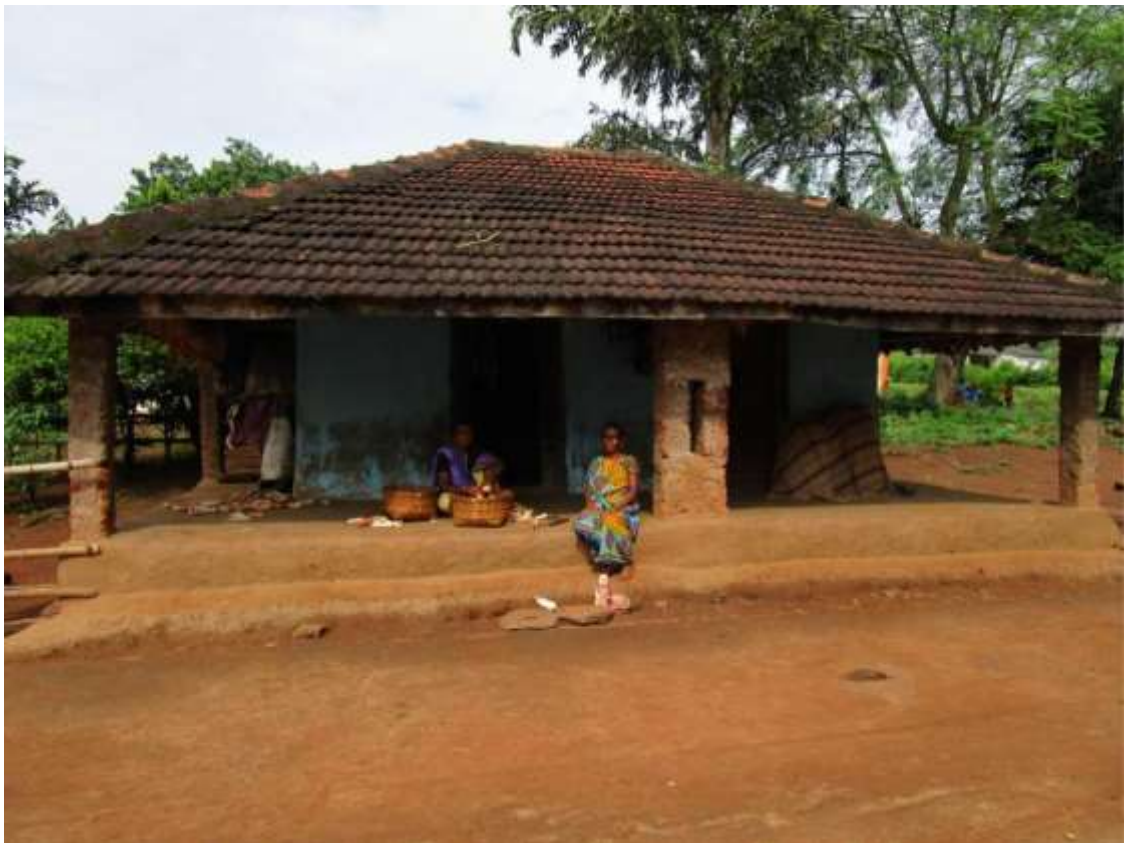
Figure 8 A tiles roofed house at Vamugedda, Chinthapalle Mandal
