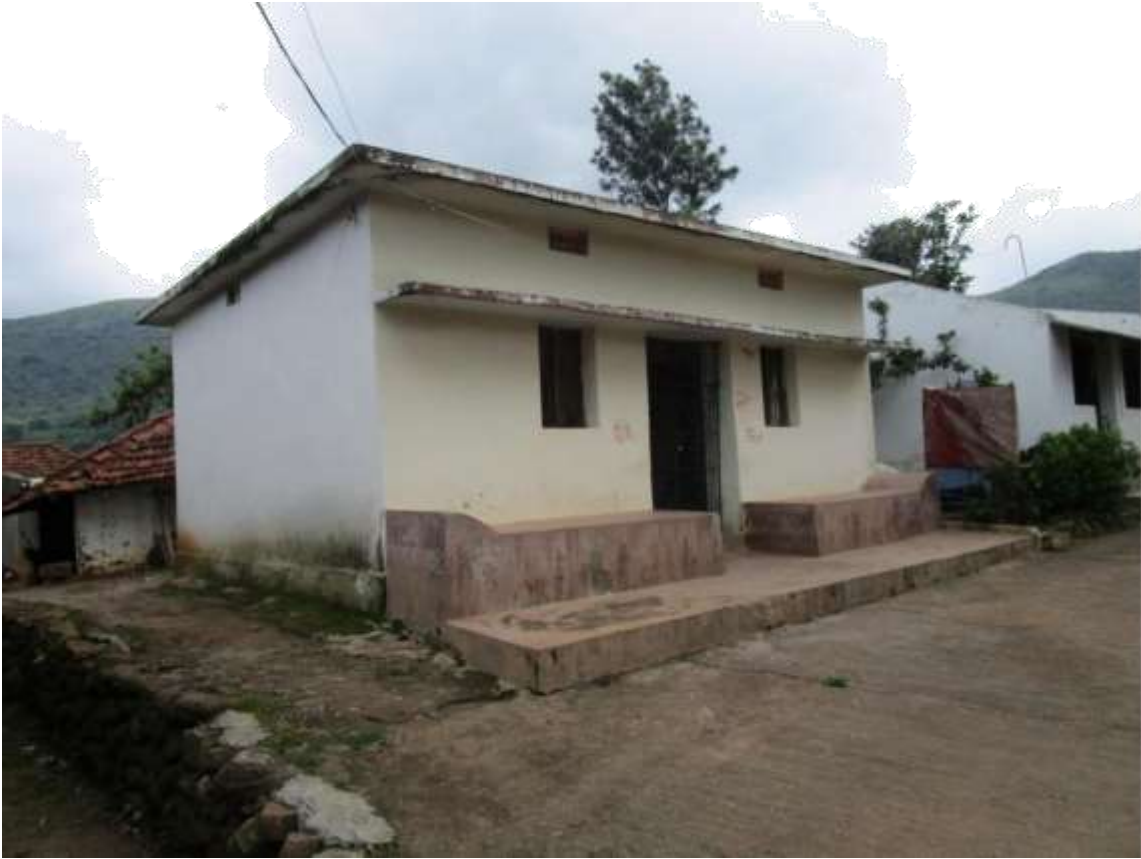
Figure 13 A RCC House at Bakuru village, HukumpetMandal
