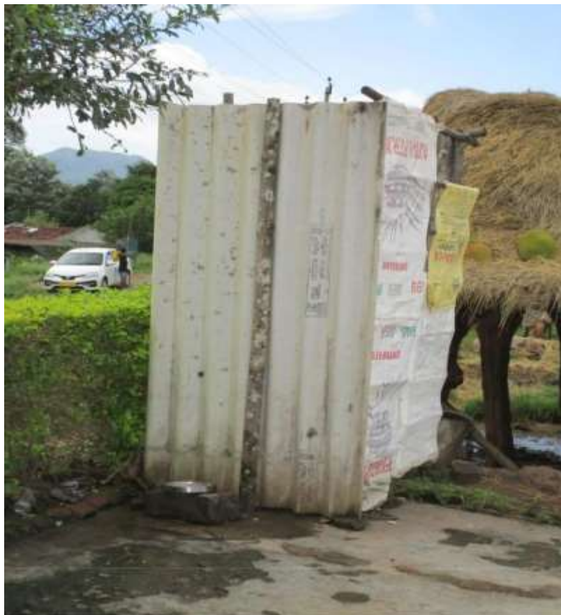
Figure 44 Bath room made with asbestos sheets outside the house
