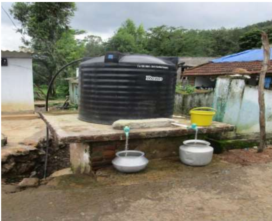
Figure 57 Protected drinking water at PathaPaderu village, Paderu Mandal
