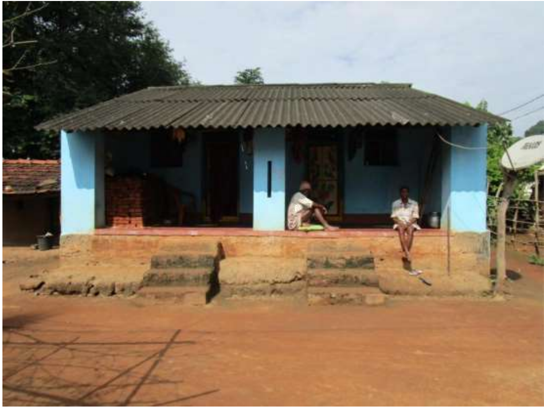
Figure 7 Asbestos sheet roofed house at Bailukunchingi, Chinthapalle Mandal
