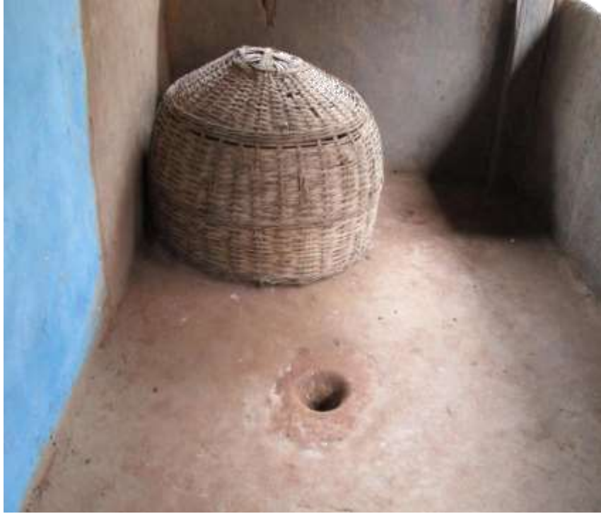
Figure 76 Pounding mill embedded in the floor
