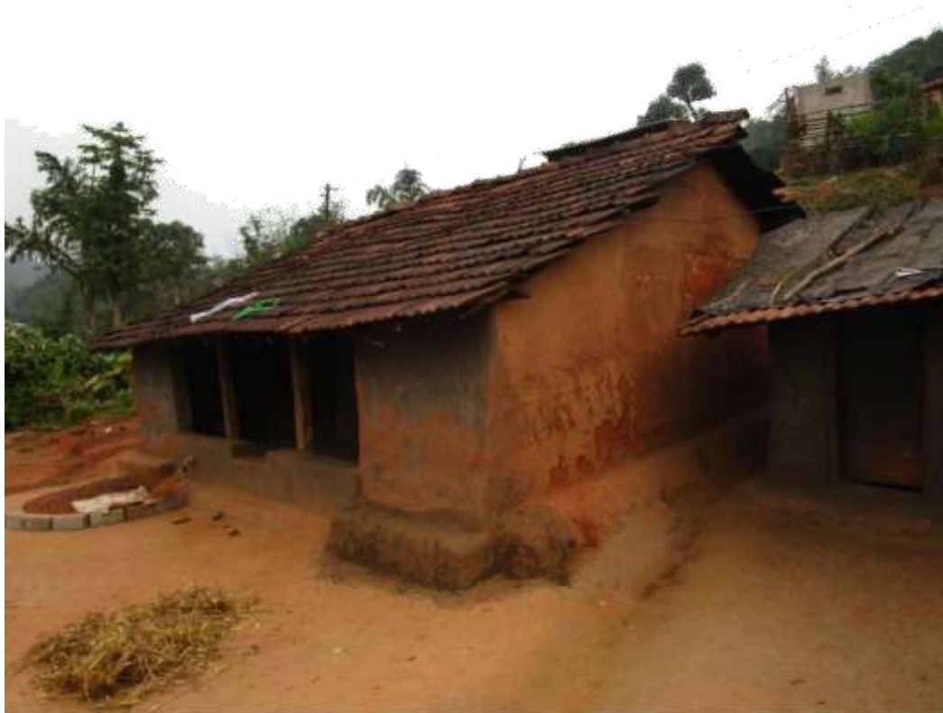
Figure 9 A tiles roofed house built with mud walls at Adaparai Goundhi, G.K.VeedhiMandal
