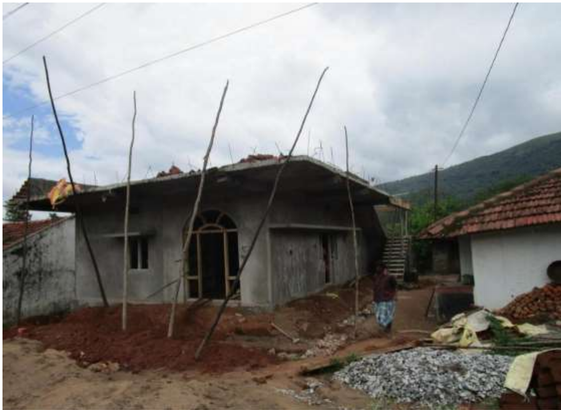
Figure 14 A RCC House Under construction at Bakuru Village, HukumpetMandal
