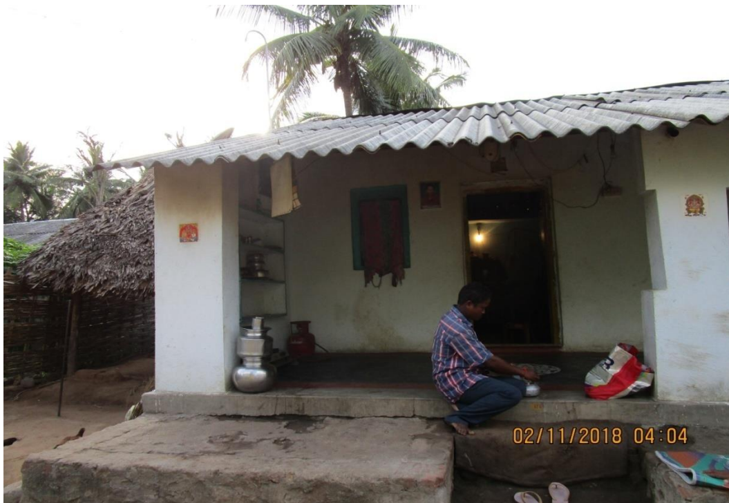
An asbestos sheet roofed house of Sokulugudem village, Rampachodavaram ITDA, East Godavari dist
