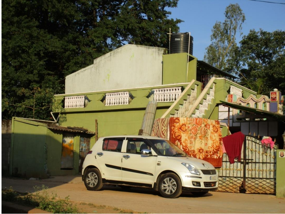
A RCC House of Konda Kapu at Yendapallivalsa, Paderu ITDA, Visakhapatnam Dist
