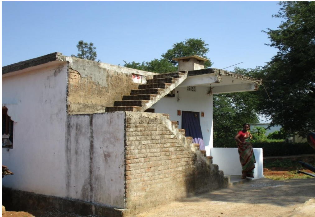
A RCC House of Konda Kapu from Araku , ITDA Paderu, Visakhapatnam, Dist
