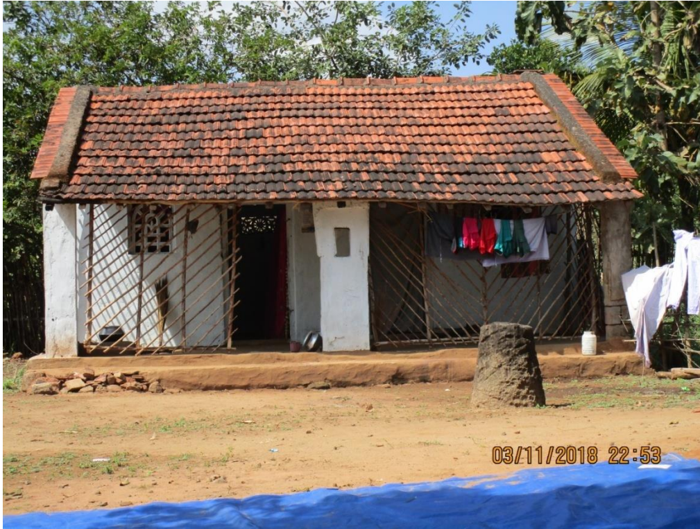
A tiled roofed house of Konda Kapu with cement plastered walls in Ramapachodavaram ITDA, East Godavari dist
