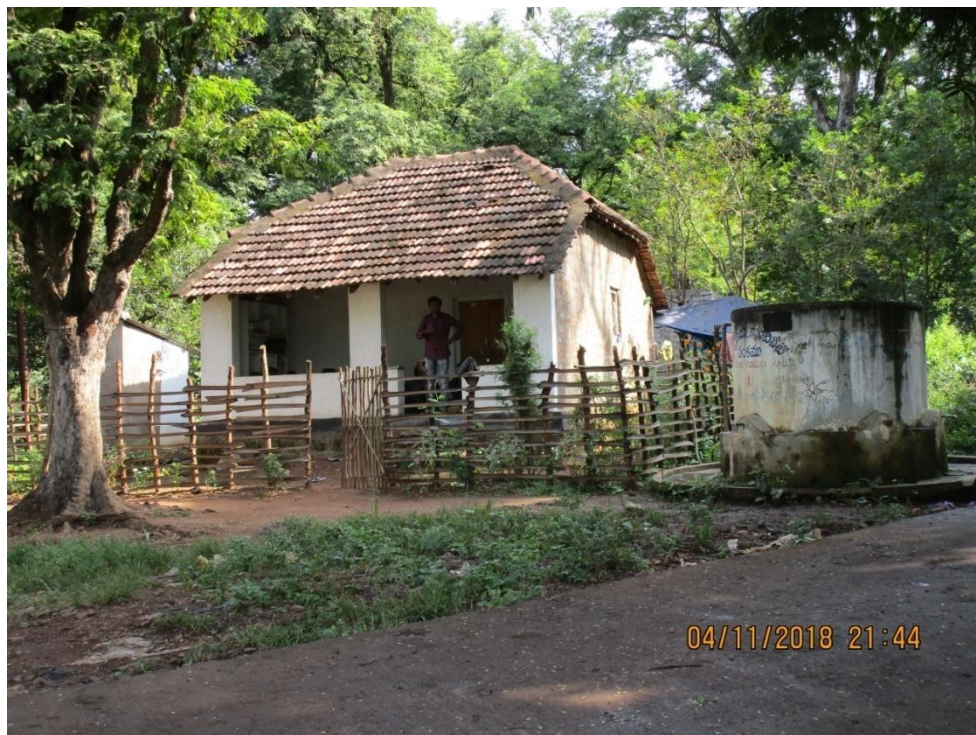
D.R. Depo, for supply of provisions and drinking water tank at Gunjugudem village, Ramapachodavaram ITDA, E.G.dist
