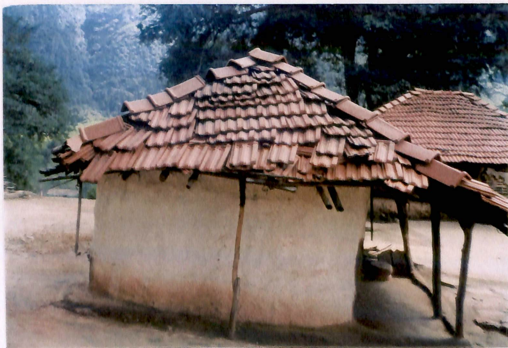
Irregular Spreading of Tiles- Katiki(V), Ananthagiri(M).
