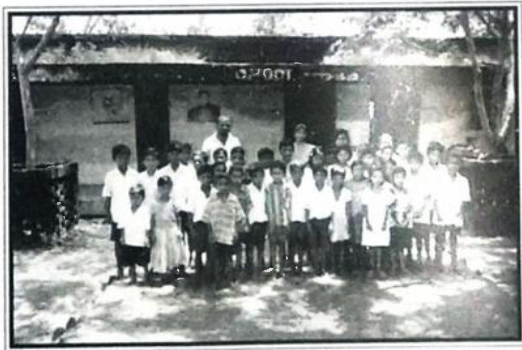
School building provided by MCL Ib Valley in Madhuban Nagar Resettlement Colony.
