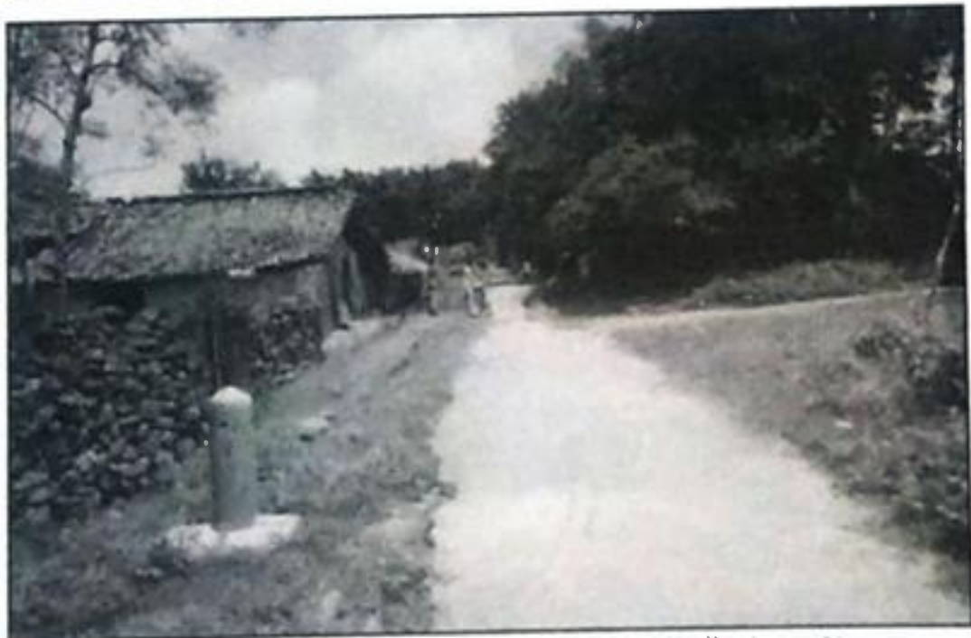
House Condition of ST household in Madhuban Nagar Resettlement Colony (MCL Ib Valley)
