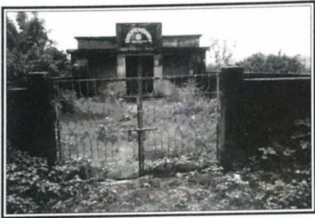
Dispensary provided by MCL Ib Valley in Madhuban Nagar Resettlement Colony.
