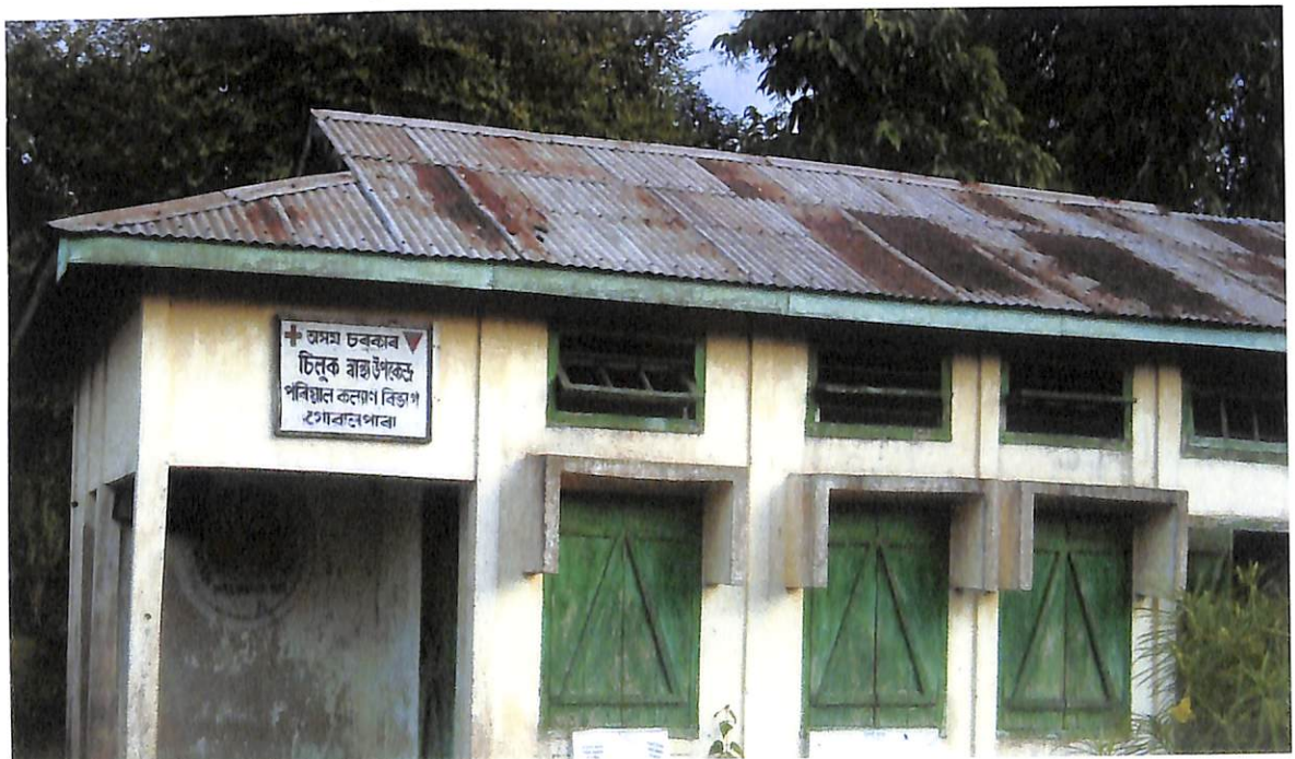
A HEALTH SUB-CENTER AT SILUK
