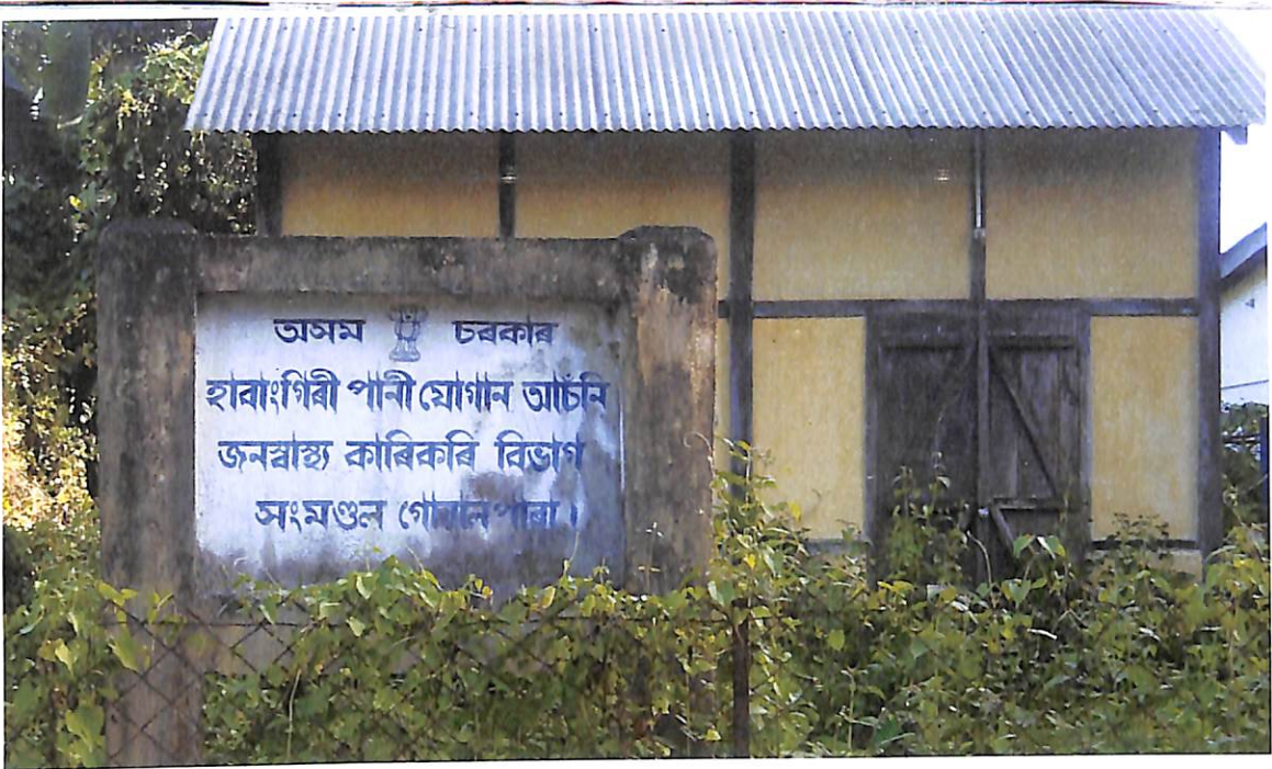
WATER SUPPLY AT HABBANGIRI
