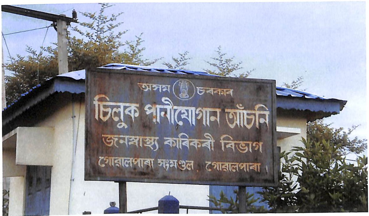
A WATER SUPPLY AT SILUK
