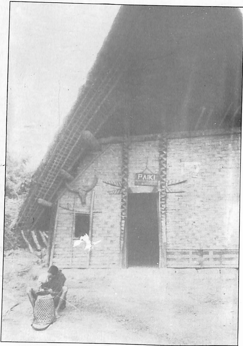
The front view of a Zeme boys' Morung.
