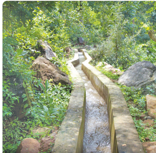
Completion of Incomplete Field Channal at Angora through SCA to TSP 2009-10
