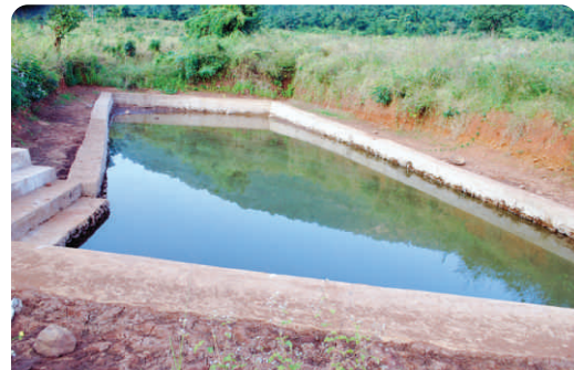
Construction of D/W at Vill-Rangaparu, G.P-Belghar, Block-Tumudibandha, Dist-Kandhamal
