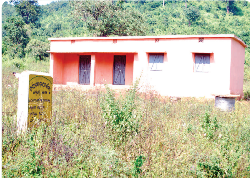
Construction of M.P.S.C. building at Vill-Madalakuna, G.P-Belghar, Block-Tumudibandha, Dist-Kandhamal
