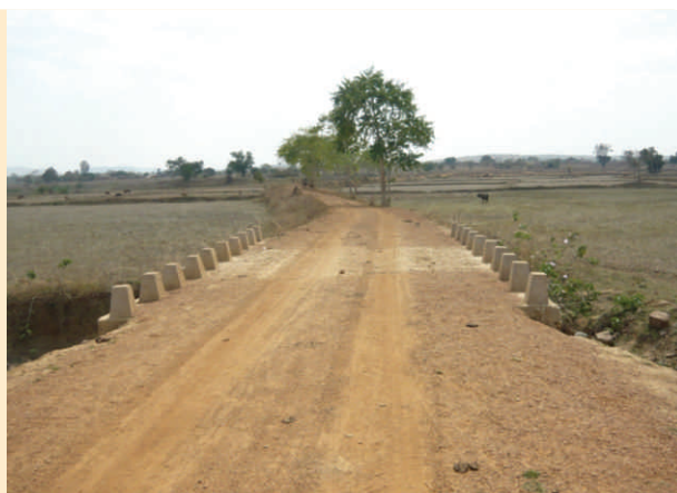
Improvement of road from Sunabeda to Junapani
