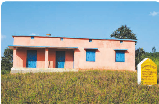
Construction of M.P.S.C at Vill-Pandamaska, G.P-Belghar,Block-Tumudibandha, Dist-Kandhamal
