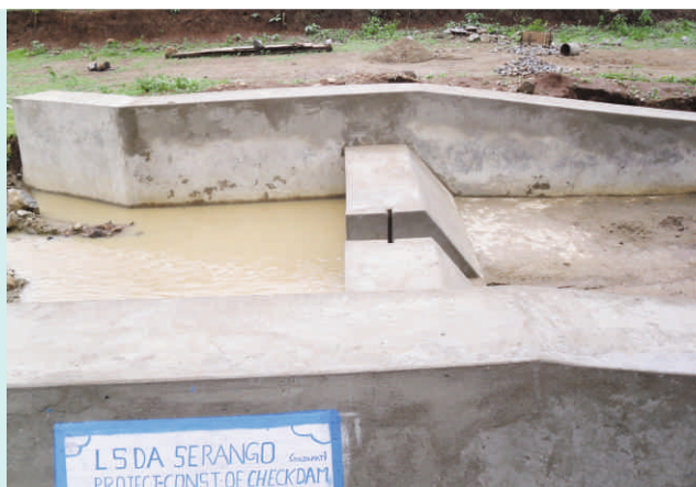
Construction of Check Dam at Kutamtal Nalla, Rudhei
