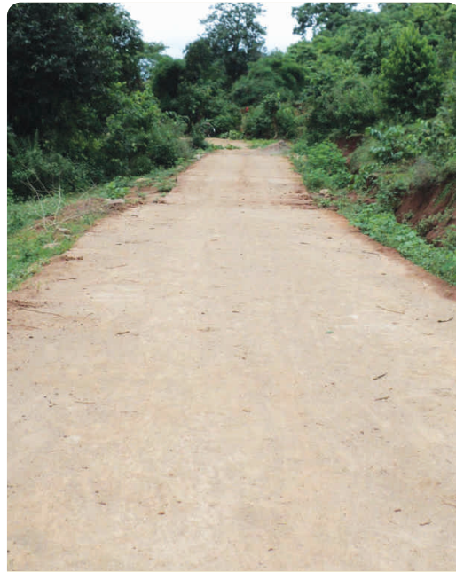
SCA to TSP CD work at Bahadapada, Chandragiri
