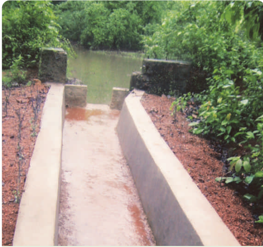
Construction of canal with D/W under CCD plan 2009-10.
