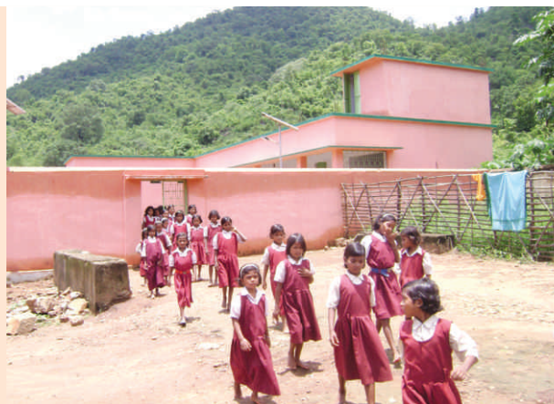
CONSTRUCTION OF ADDITIONAL HOSTEL ROOM AT EDUCATIONAL COMPLEX, SAKATA
