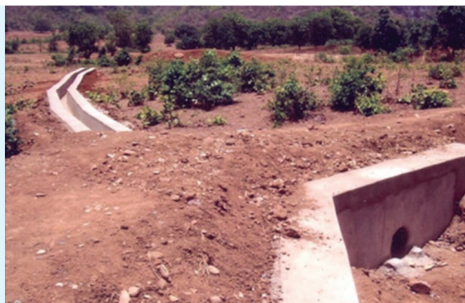
CONSTRUCTION OF CANAL SYSTEM OF BAGHIANALLA WHS
