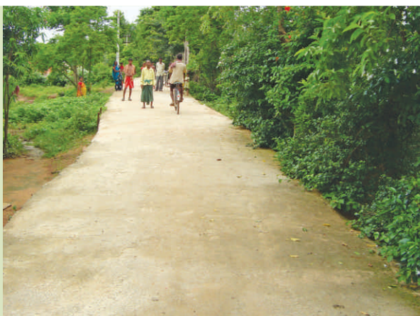
Construction of CC Road and Culvert at Patharnesa under Suliapada Block
